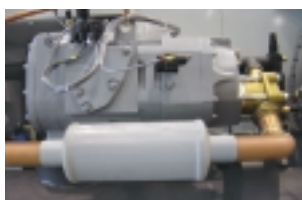
Muffler on Discharge Pipe
